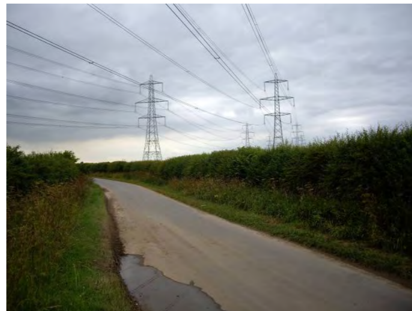
Photographs showing close synchronised parallel overhead lines with L6 and L2 tower designs
