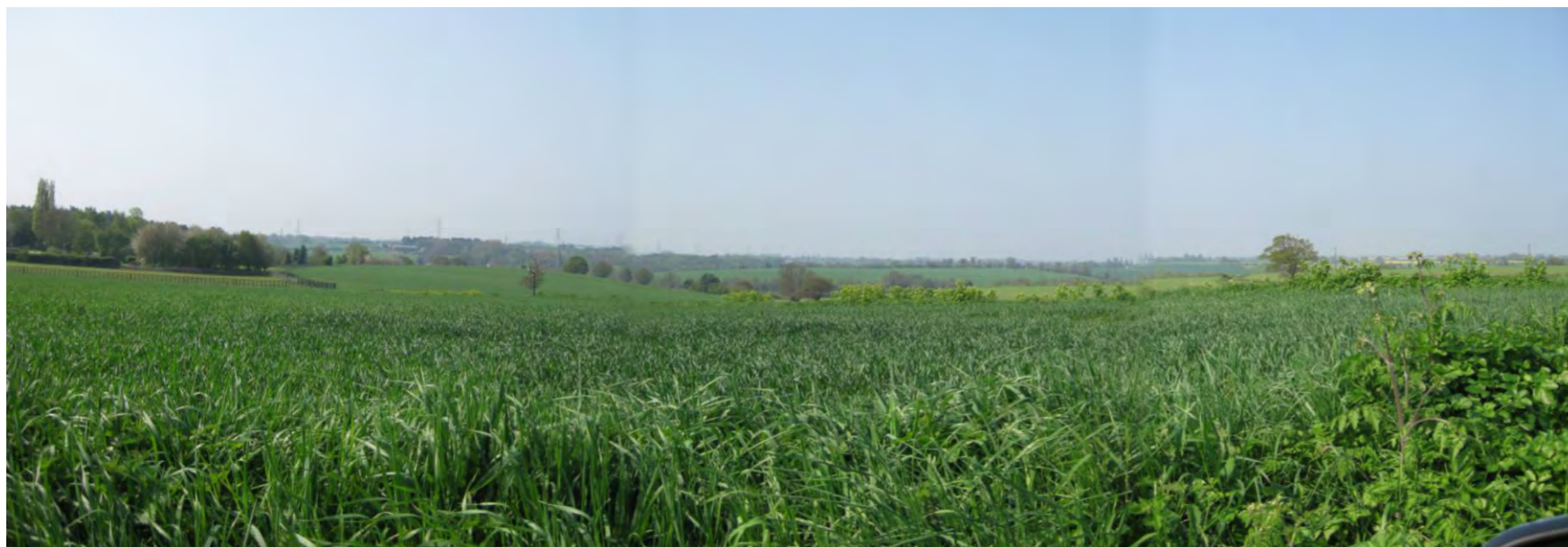
Photographs to show the existing 132kV and 400kV overhead lines in the river valleys
